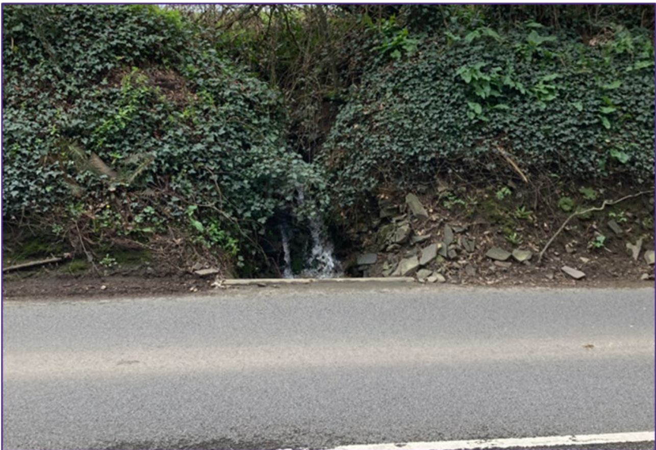
Plate 1.5: Culvert which runs under the A386
